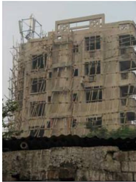
Picture 9 Constructing Narkeldanga
