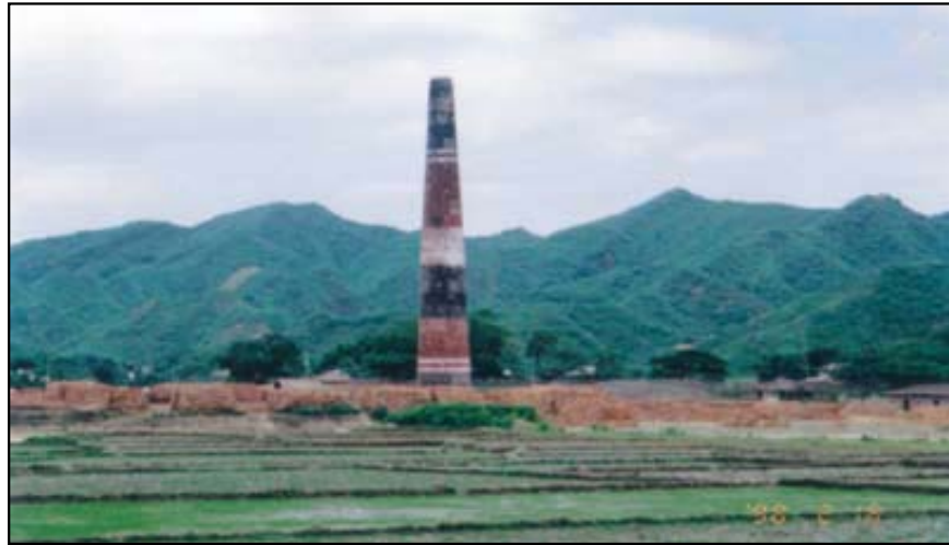
Plate 5: A typical brickfield inside the game reserve in Ledha.
